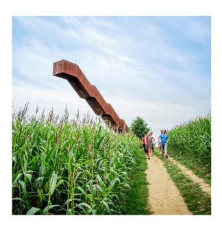
The floating staircase is made of stainless COR-TEN steel, its colour reminiscent of its ironstone heritage. It stands at over 11 m high and is more than 20 m long. It's at the top of one of the Hageland's highest locations, an inlier around 80 m high, that you'll find this look-out staircase.
